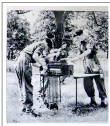
Setting up a field telephone exchange (Photo = The Sphere)
